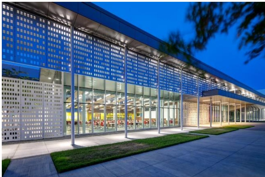
Data center Fort Worth (EUA)
